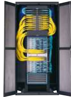
Net-Access™ N-Type Cabinet with Cisco^ Nexus 7018 Extension Kit Installed
